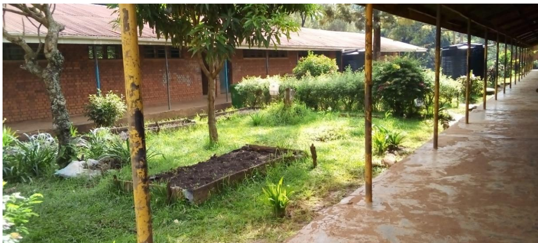
Figure 44: Image showing the 2 classroom blocks planned around a quadrangle with the passages facing inwards.
