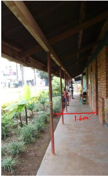
Figure 43: Image showing passage at administration block.
