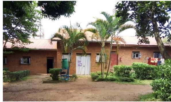
Figure 50: Image showing the exterior of the boy's dormitory
