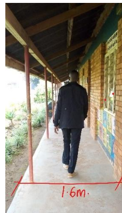
Figure 67: Passage at the administration block
