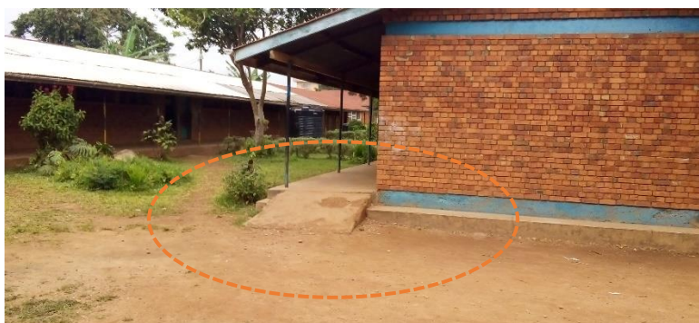
Figure 64: image showing a ramp leading to the classrooms.
