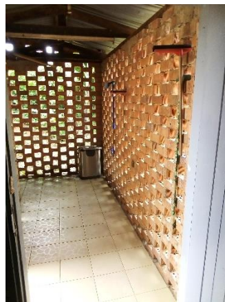
Figure 58: Perforated brick wall in the girls toilet allows for sensory reach
