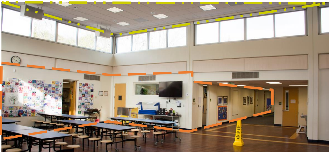
Figure 33: Atlanta speech school, cafeteria showing acoustic ceiling tiles and soft board walling (Hauan 2017).
