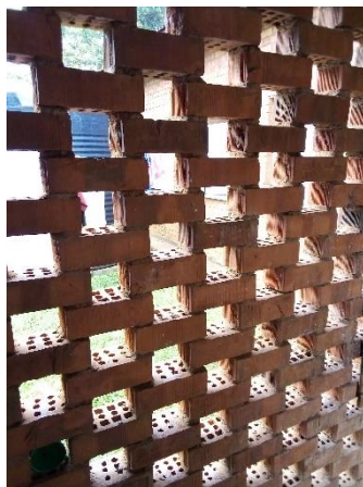
Figure 58: Perforated brick wall in the girls toilet allows for sensory reach
