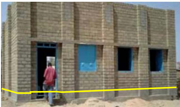
Figure 4-4: Showing the raised plinth level.
