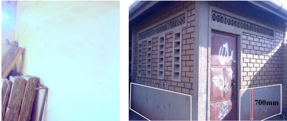
Figure 4-11: Showing Plastered interior walls and exterior region respectively.
