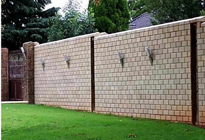
Figure 5-8: Boundary wall with interlocking block (Source: Hydraform)
