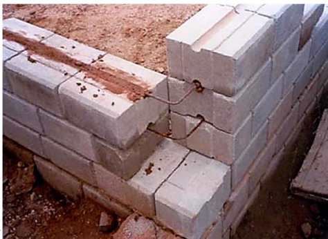
Figure 5-9: Bonding corner edges with Steel bars.
