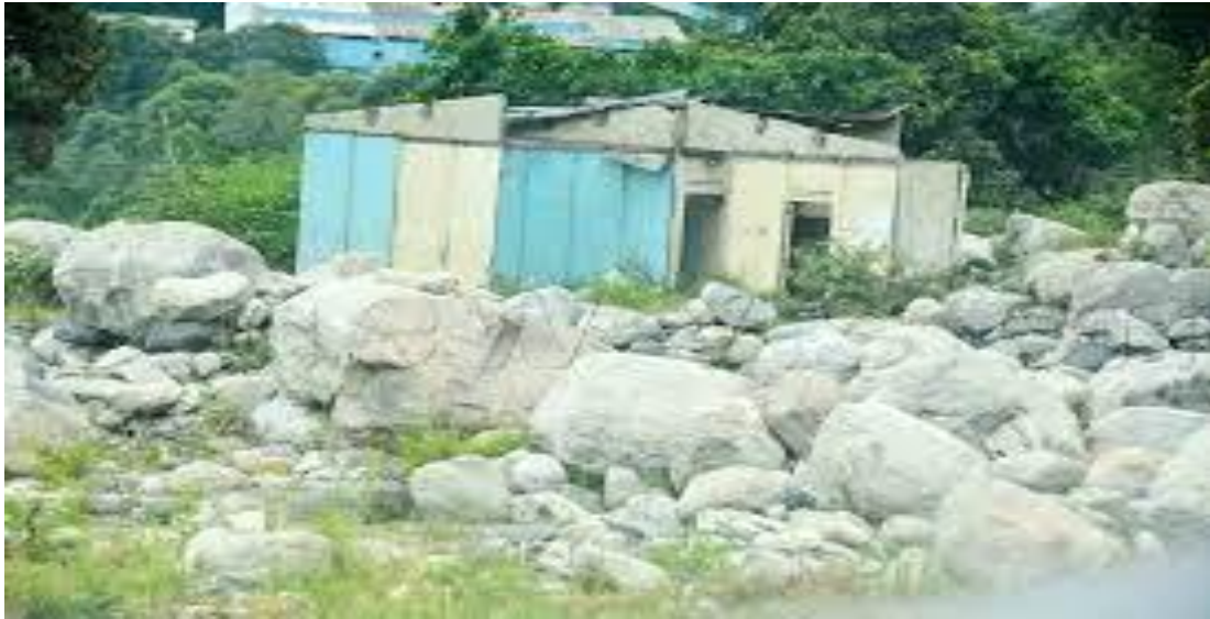
The above photography 3 show s destroyed house in the Nyamwamba river where huge stones brought by the river were left deposited outside the house in Nyamwamba river valley.
