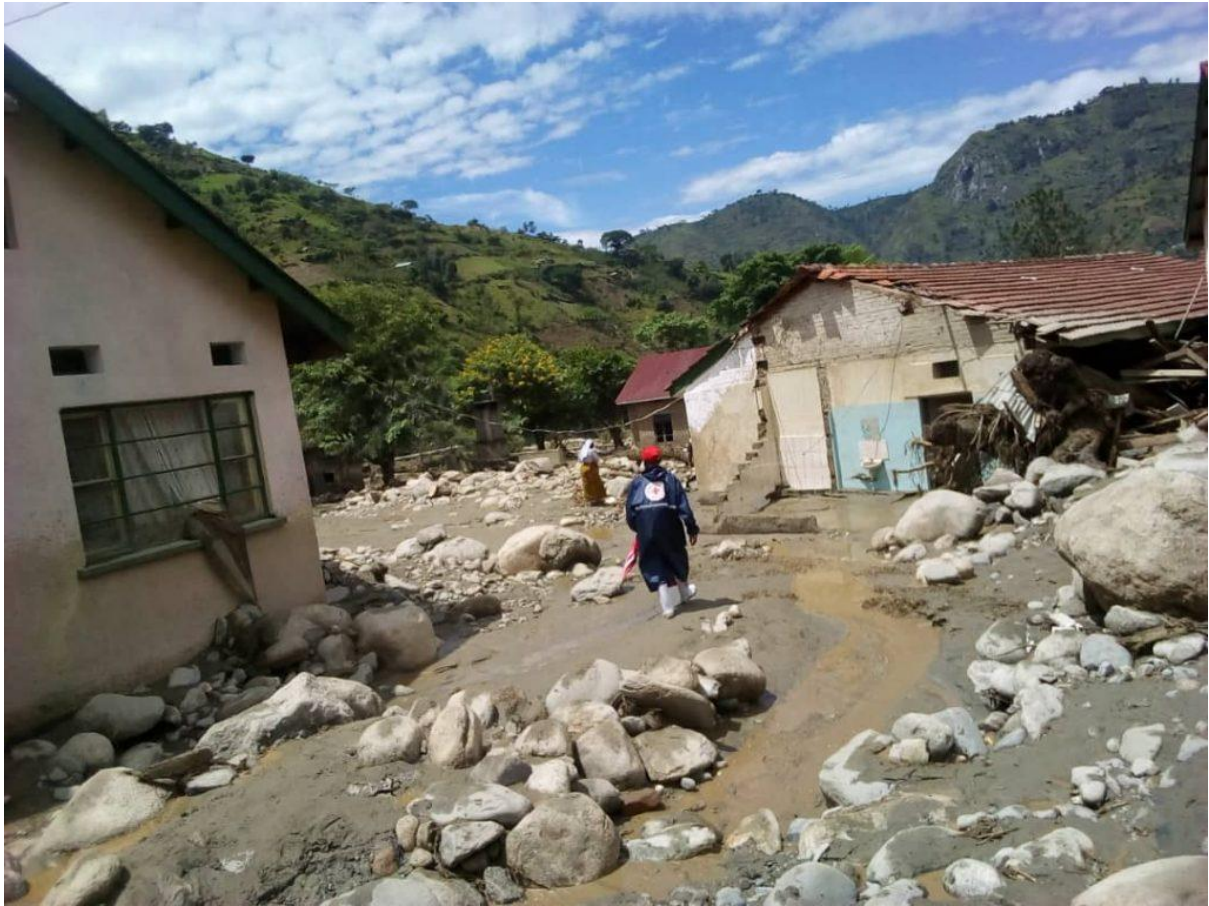
Houses destroyed in 2020 by violent floods (File Photo by RED CROSS)
