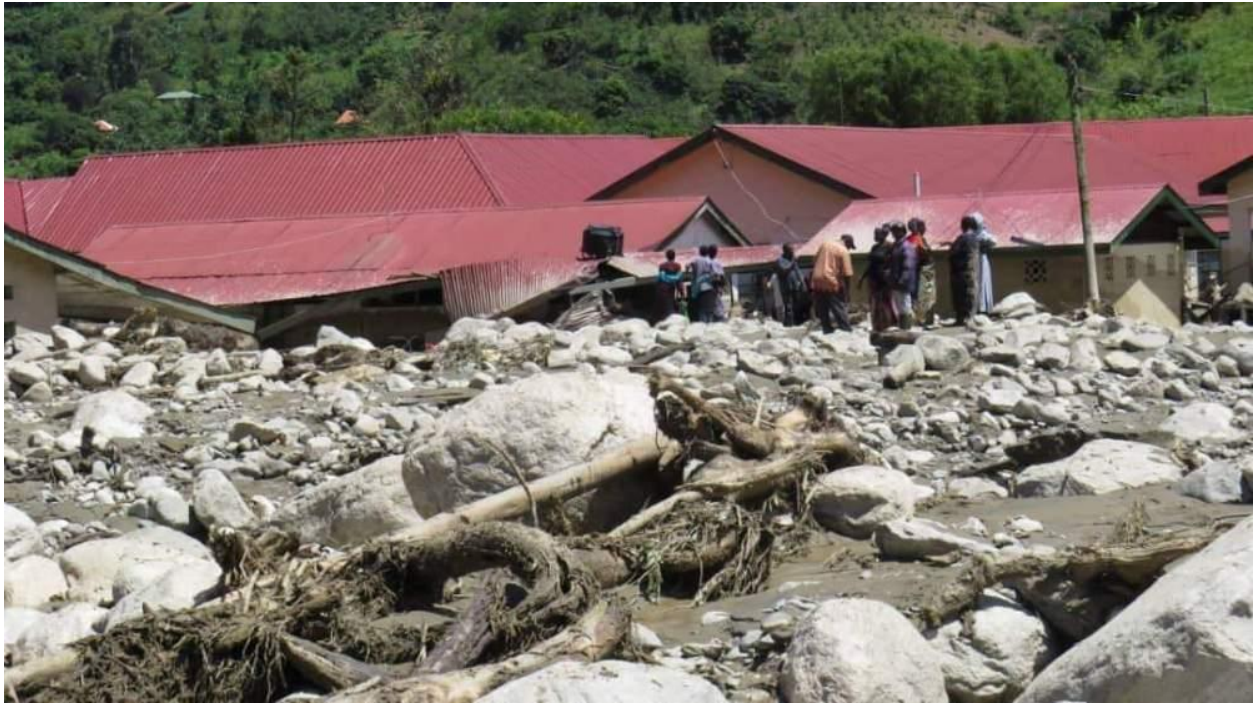
Houses destroyed in 2020 by violent floods in kasese municipality (file photo)
