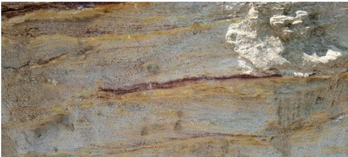
Figure 3. 5: Sand layers encountered along Kibuku Road Cut
