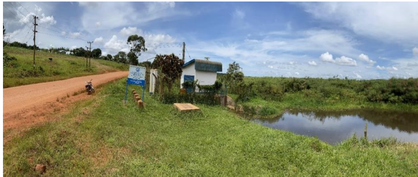
Figure 4-1: Unprotected intake at Kiyanja Swamp
