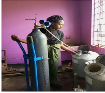
Figure A-3- 1: Purging using nitrogen 1
