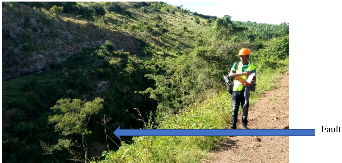
Figure 24: A fault zone with NE-SW trend evidenced by a linear pattern of vegetation especially in valleys and nearly straight scarps that trend some-what downhill
