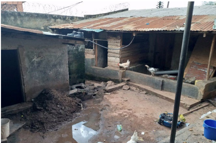
Figure 19: Centralized Arrangement of Low-Income Houses. (Source: Author).
