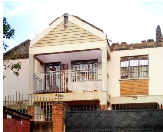
Figure 23: Half Demolished House
