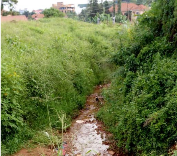
Figure 32:Kabanyanya Drainage Channel (Source: Author)
