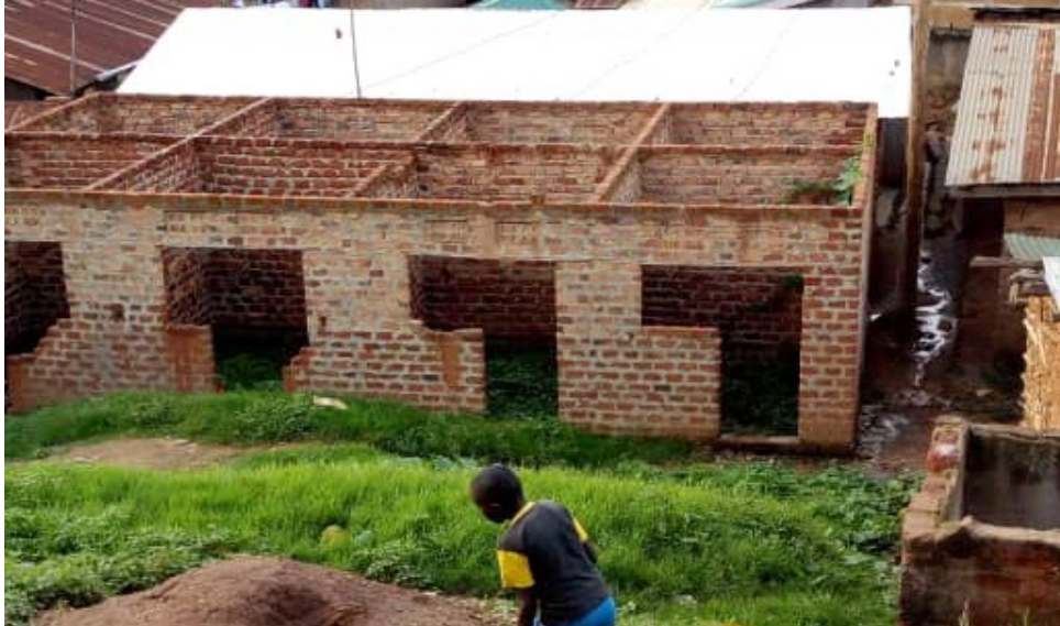
Figure 24: Unfinished Vacant Houses. (Source: Author)
