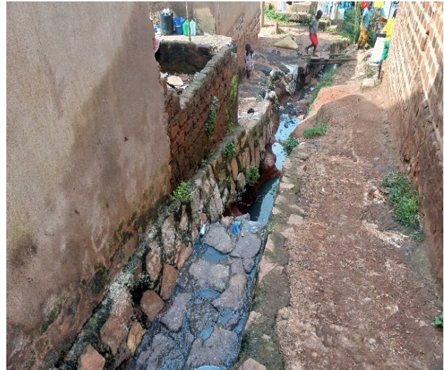
Figure 32:Open Drainage Channel (Source: Author)
