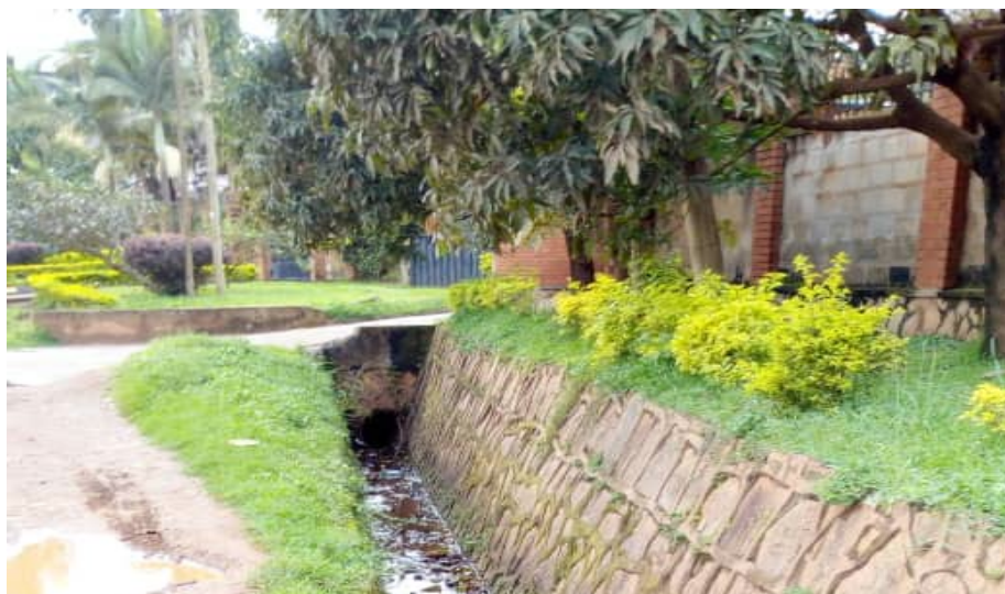
Figure 30: Open Drainage Channel along Naguru-Katale Lane. (Source: Author)
