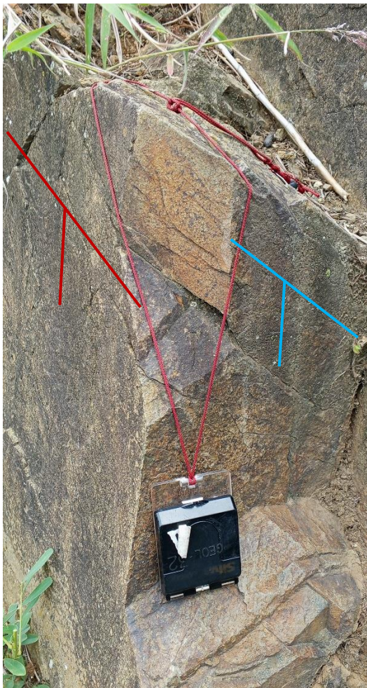
Figure 24. Shows are highly Jointed rock outcrop with various joint sets.
