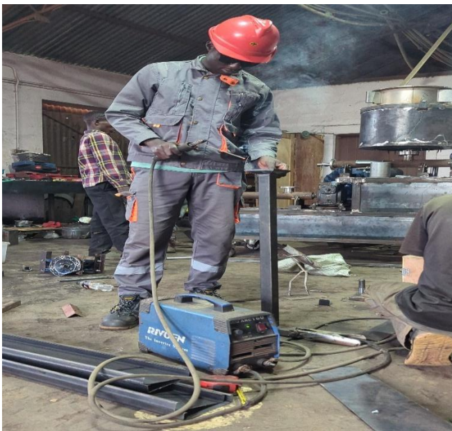
Figure 11: Welding of the planter
