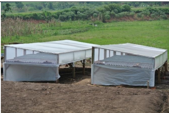
Figure 2-1 Static bed box solar dryers (Kiggundu 2016)
