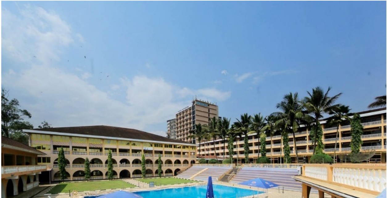
Figure 18 Image showing the Africana Convention Centre and Nile Hall on the premises of Hotel Africana
