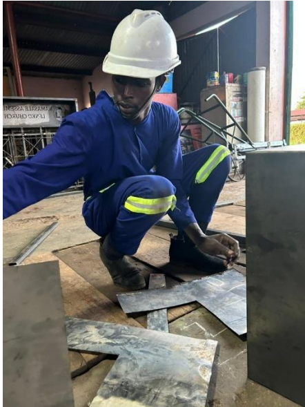
Figure 28: Preparing the mild steel material for the outer cabin
