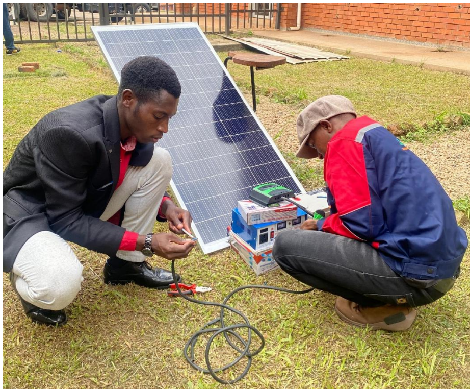
Figure 18: Solar electrical assembly – PV panel, MPPT controller, LiFePO 4 battery
