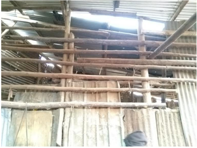
Figure 36: Iron sheets and poles used as walling material. Source: Author, 2021.
