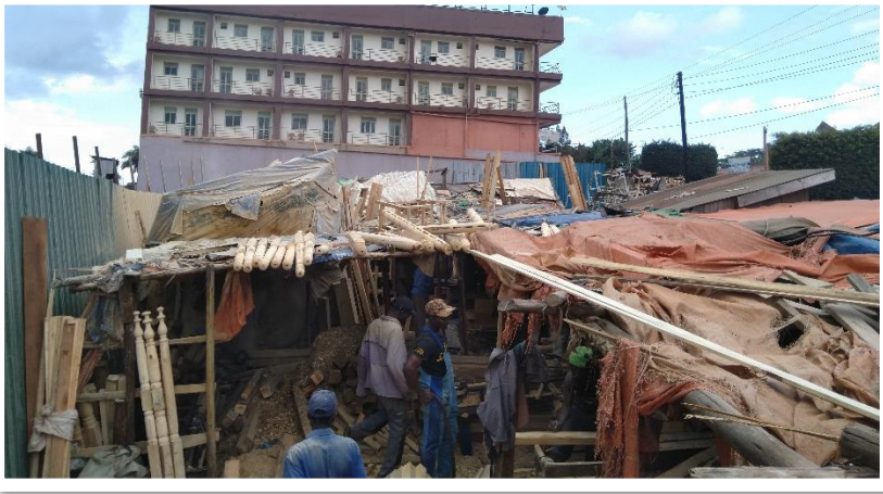
Figure 9: A display of different colours from the different roofing materials(Source: Author, 2021).
