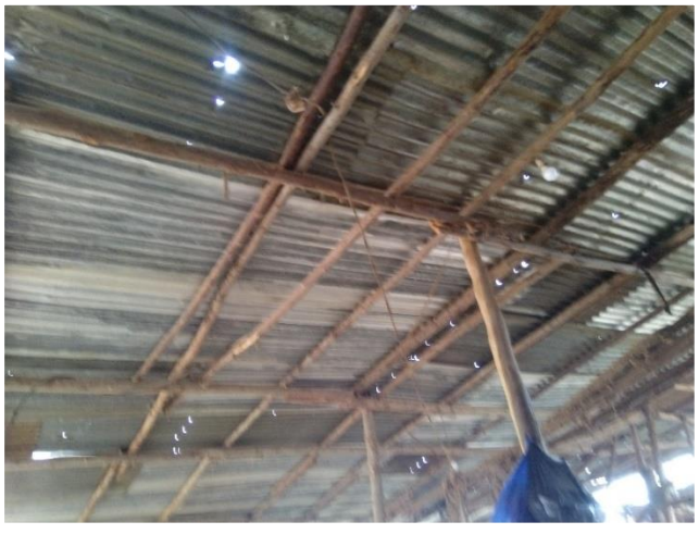
Figure 35: The roof system. Source: Author, 2021.
