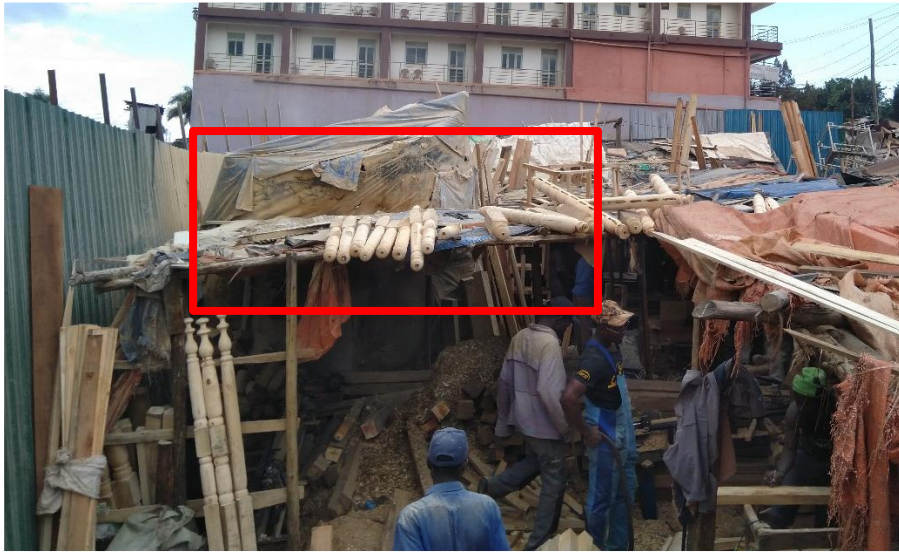
Figure 14: Bed components temporarily kept on the roof before assembly. Source: Author, 2021.
